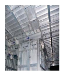
The combination of pin-wedge and bolt-nut connections allow easy connection of accessories such as guardrail brackets, aligner brackets and plumbing brace brackets.
