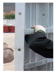
Aluma EasySet® offers lightweight panels with stiffeners that provide two functions: (1) Structural strength and (2) practicality. Panels can be easily maneuvered via the stiffeners.
